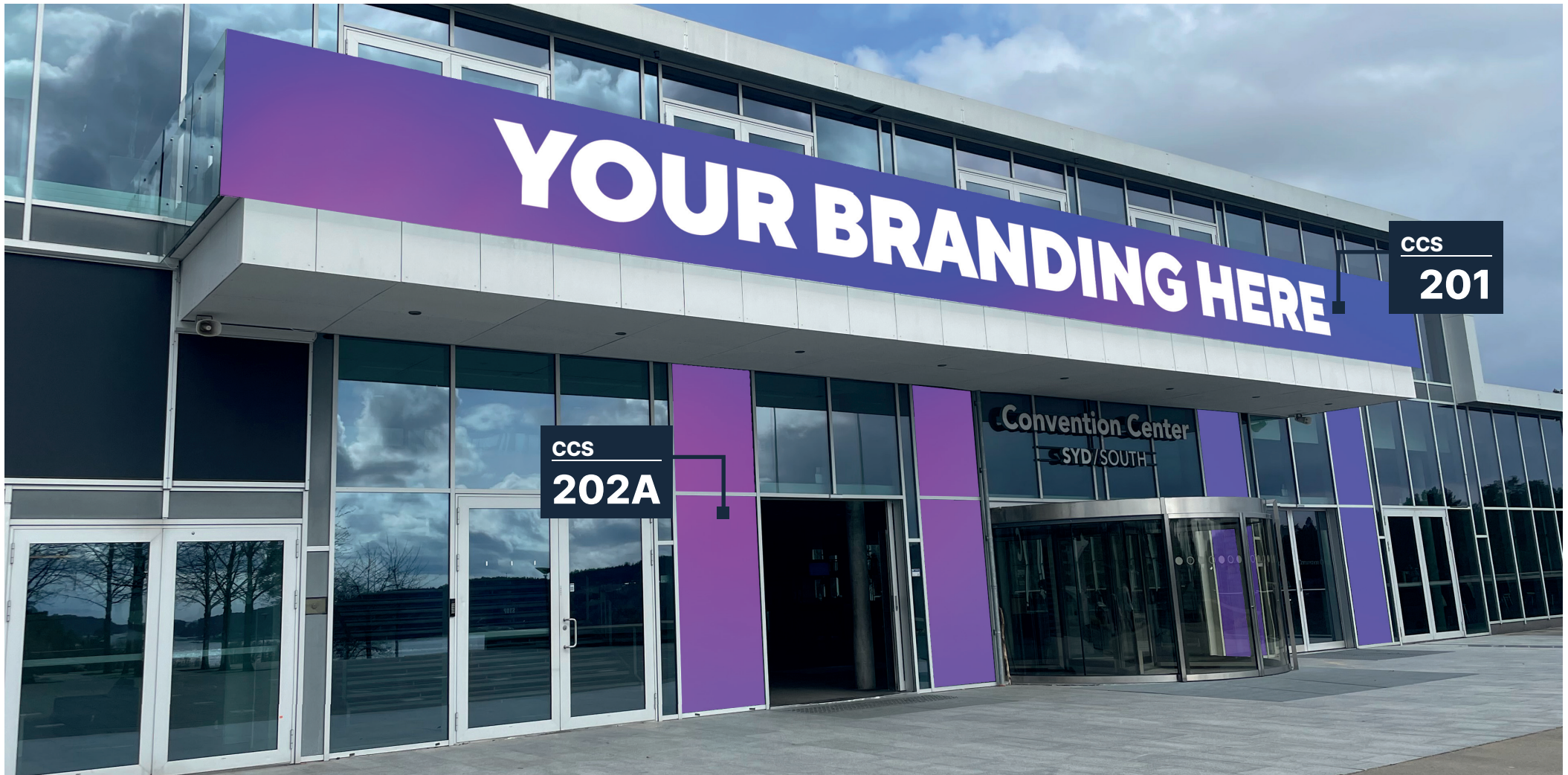
CCS 201: Glass railing above the main entrance to CCS
