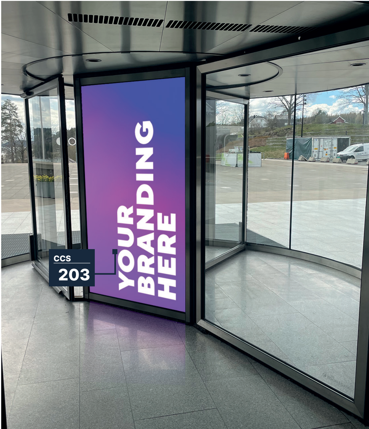
CCS 203: Glass inside Revolving Entrance at CCS
