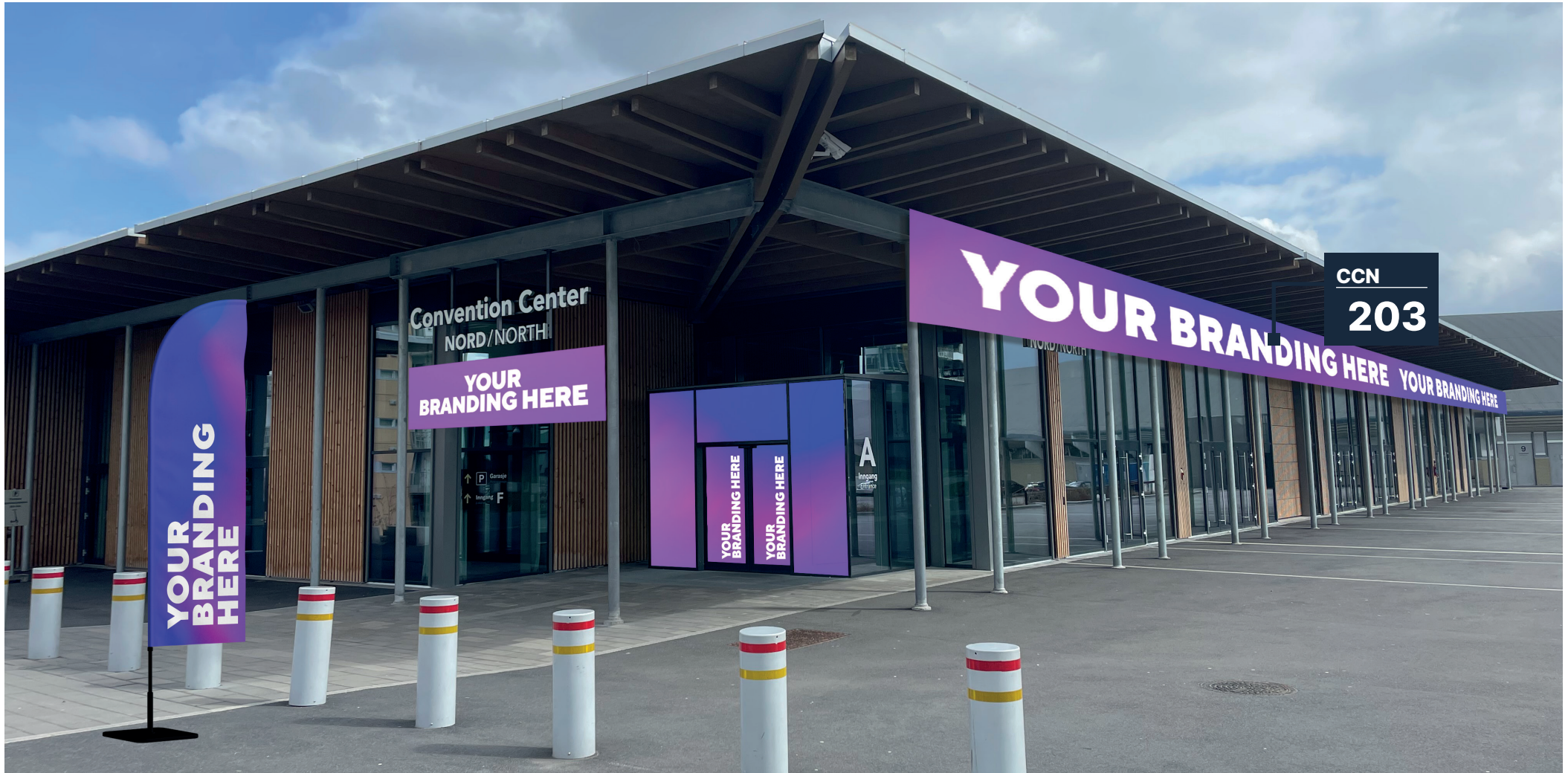
CCN 203: Hanging banner along the length of CCN, in front of the facade
